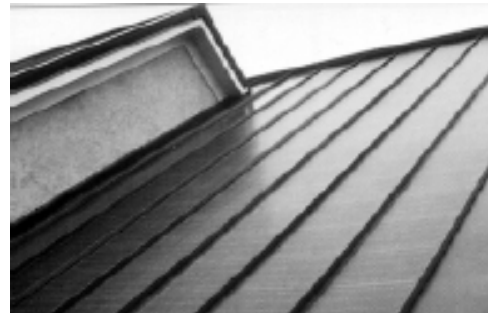
Figure 12: Example of Standing Seam Roof ( www.cisolar.com )
