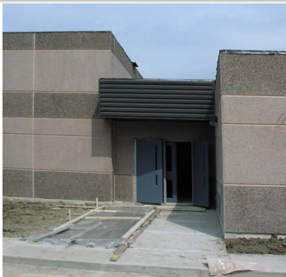
Figure 21: Example of Precast Masonry School Building ( www.cpci.ca )
